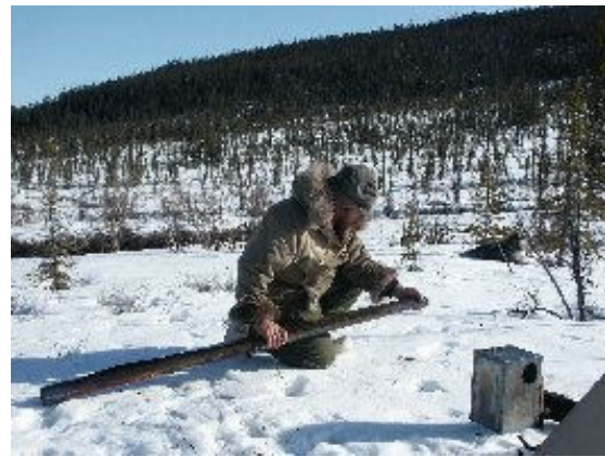
Rolling the stovepipe into shape
